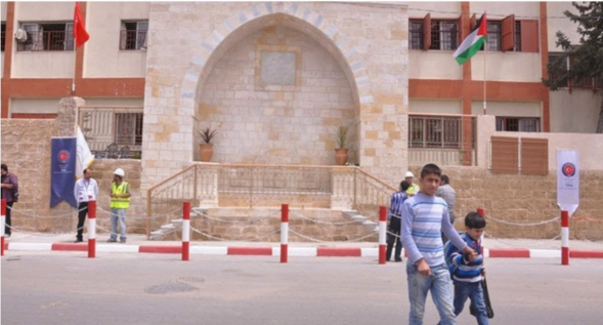
Figure 4: The Abdülhamid (Rifa'iyya) Fountain in Gaza. Detail from an aerial photo of c. 1917, showing the fountain from behind, opposite the municipality building. Photograph of 2017, showing the fountain's façade after recent renovation works.
