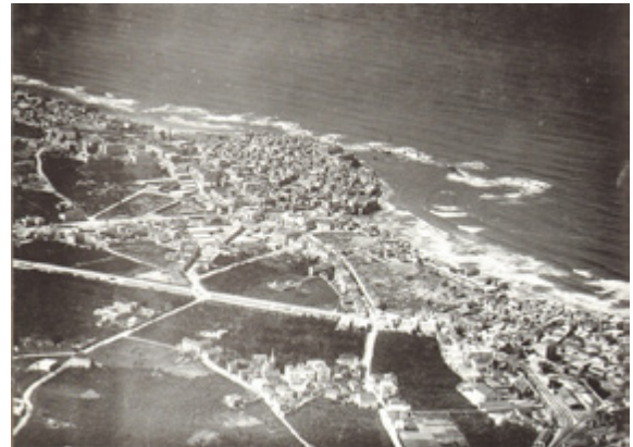
Figure 5: Aerial Photograph of Jaffa in 1917. Note the Old City and the harbor in the center and the beginnings of the ‘Ajami neighborhood south of the harbor. On the other side, the road leads to the northeast (towards Nablus) with Bustrus Street, which is intersected by Jamal Paşa Boulevard (constructed during World War I), and somewhat farther along to the German Colony (note the church tower in the picture). Gustav Dalman, Hundert deutsche Fliegerbilder aus Palästina (Gütersloh: Bertelsmann, 1925), p. 77.
