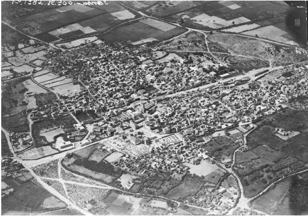
Figure 2: An Aerial View of the Government Compound Area from the South, c. 1917. Source: CZA, PHG/1065479. Aerial photograph of Gaza, c. 1917.
