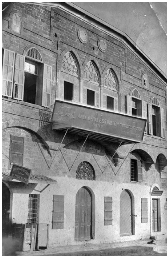
Figure 10: The 'Isas' House on 'Ajami Street. A floor was rented out to the Zionist Anglo Palestine Bank from 1903 to 1922/23. Photograph from the Mandate period (courtesy of Samuel Giler).
