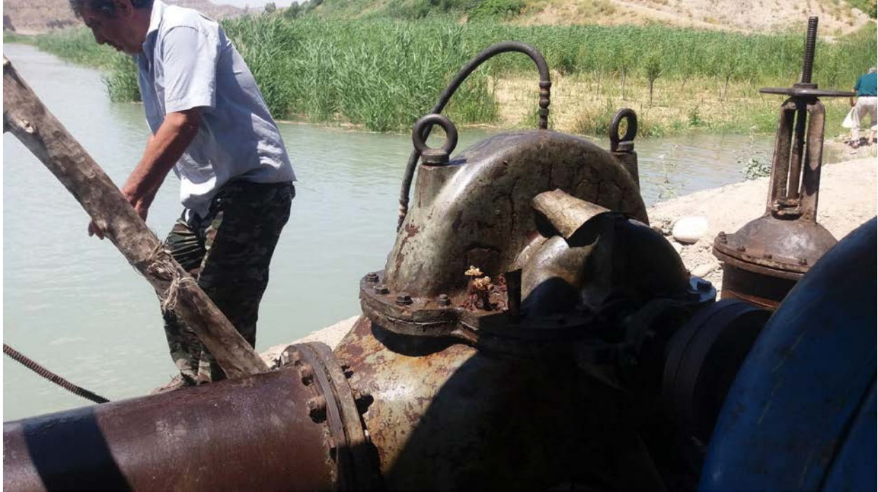
Figure 4.1. Ahmatjan Aba on the Naryn River fixing the water motor to distribute water for irrigation. Source: Baialieva, Tendik village 2018.
