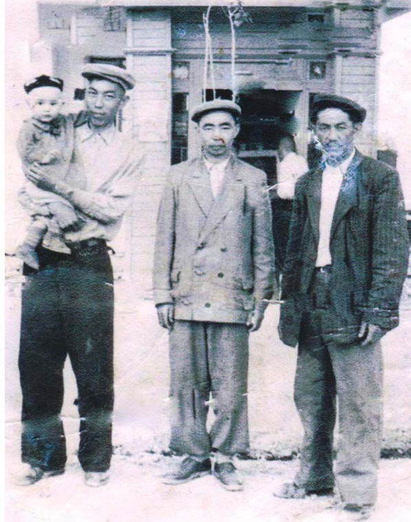
Figure 3.5. Construction workers at the beer shop in Shamaldy-Sai in 1959. From the left: my grandfather Turaly holding my mother, uncle Makambai and uncle Orozbai. Source: Baialieva's family album.
