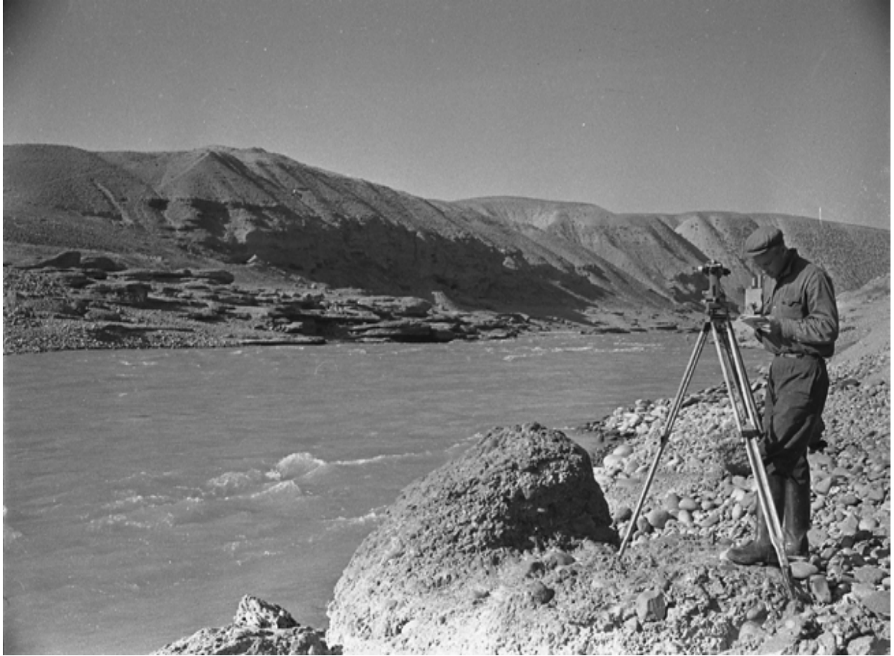
Figure 3.4. Laying the diversion channel route on the Naryn river for the future Uch-Kurgan hydropower plant. Uzbek SSR. 1957. Source: Photograph No 0-42870, TsGA KFFD RUz.
