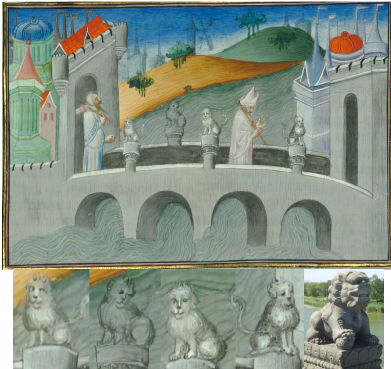
Figure 3: The Pulisanghin Bridge, with Details of the Marble Lions Adorning the Railings
