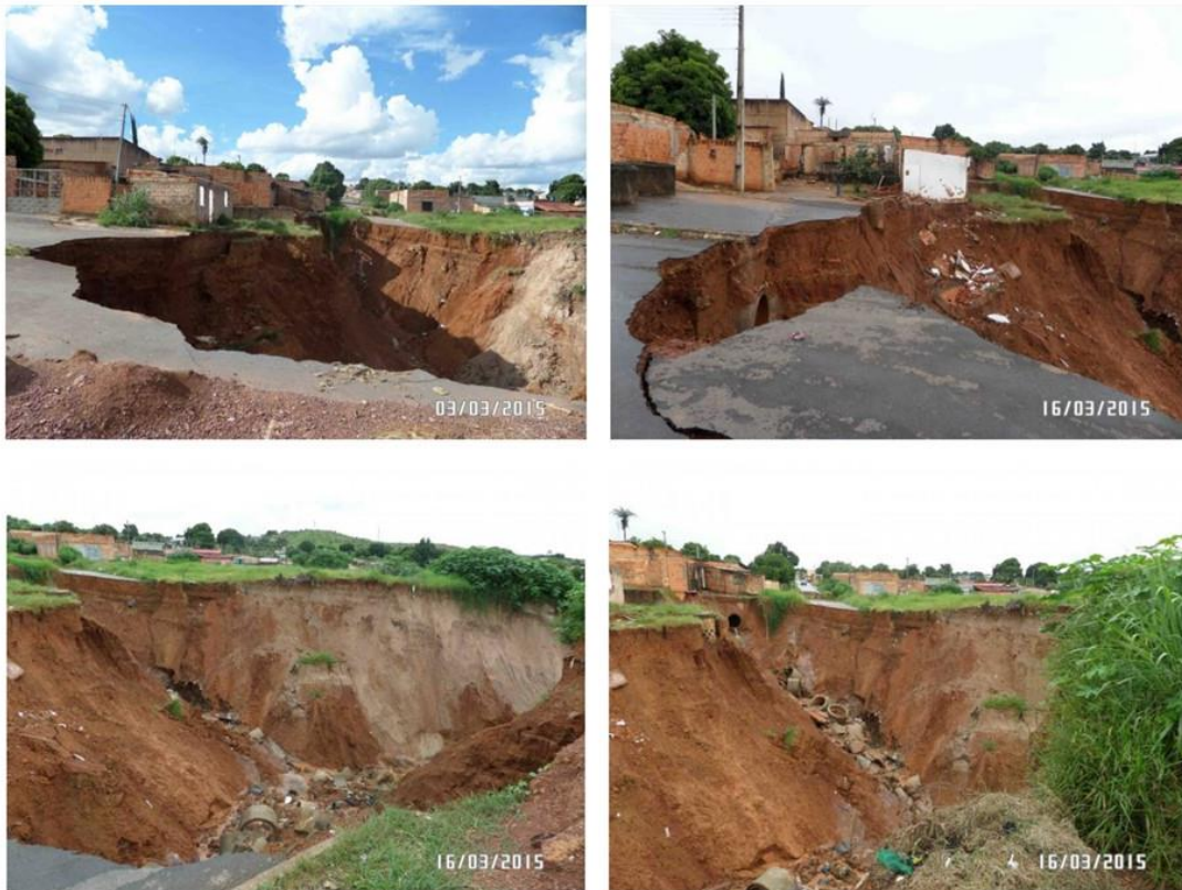
Figure 10. Destruction of public structures and residences in the municipality of Novo Gama, state of Goiás (Pimenta 2015). (Source: S2ID system reports).
