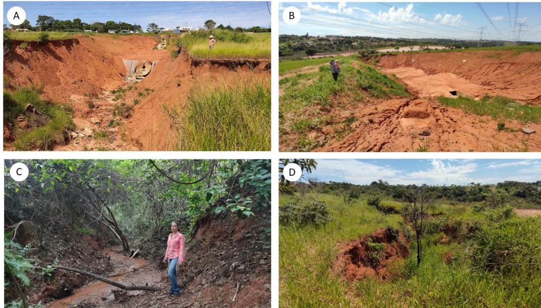
Figure 19. a) top view of ravine 5, the implemented works already have some of their functionality damaged, b) top view of ravine 5, where it is possible to observe grooves demonstrating the concentration of surface runoff into the ravine channel; c) gully 1, which shows water flow in the channel and vegetation composed of trees in the surroundings; d) ravine 2, with pasture and small trees inside and around the channel, indicating stability of the feature.
