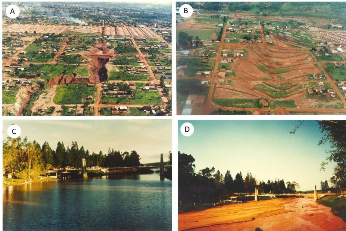
Figure 8. A) gully of Parque Bauru in 1993; B) emergency works to mitigate erosion; C) Bauru Country Club dam before the development of erosion; D) silting of the Bauru Country Club dam due to the development of erosion upstream in 1993 (Photos: Nariaqui Cavaguti).
