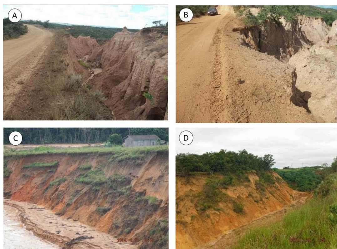
Figure 5. Examples of gullies and ravines in Brazil. A and B: Rural roads affected by erosion in Tiros, Minas Gerais state (Longe 2014); C and D: residence close to erosion and the Cascalheira stream where water is collected for public supply, municipality of Comodoro, state of Mato Grosso (dos Santos 2014) (Source: S2ID system reports).
