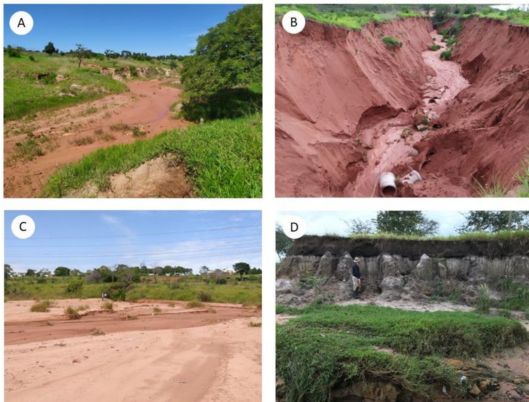
Figure 3. A) Erosion process at the valley bottom, where the lowering of the channel upstream and the silting and drying of wetlands downstream occur; B) ravine at Quinta da Bela Olinda, developed due to problems in stormwater sewers; C) silted-up area in the region of Quinta da Bela Olinda; D) soil profile, indicating lowering of the channel and drying of wetlands.
