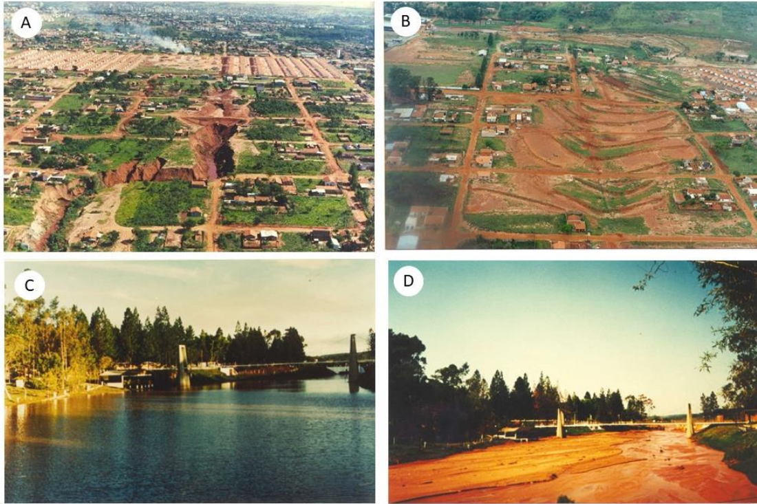
Figure 20. A) gully of Parque Bauru in 1993; B) emergency works to mitigate erosion; C) Bauru Country Club dam before the development of erosion; D) silting of the Bauru Country Club dam due to the development of erosion upstream in 1993 (Photos: Nariaqui Cavaguti).
