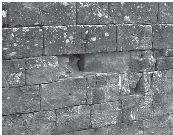
Fig. 5 A section of Wall IX N (Athena Temenos) near the Troy VI Northeast Bastion, showing the saw-cut mosaic infill; the »windows« show the original fabric behind; note mason's marks in original face blocks. Provided by the author.
