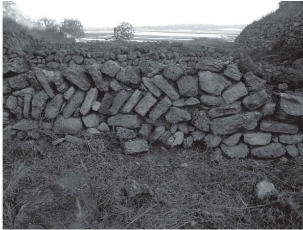
Fig. 3 A top treatment of a Troy I wall in the northern Schliemann trench, with the tile separation joint (2008); historic photos were used to re-create the typical »herringbone« technique. Provided by the author.
