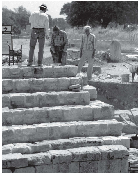
Fig. 7 The Odeion during stabilization in 1993. BW 93/076– 30 to 31.
