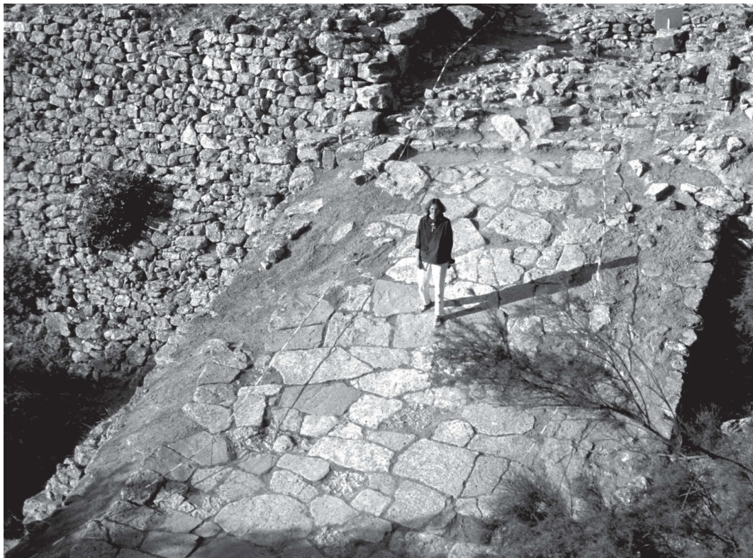
Fig. 1 The condition of the Troy II Ramp at Gate FM in 1992, before stabilization. BW 92/101-10
