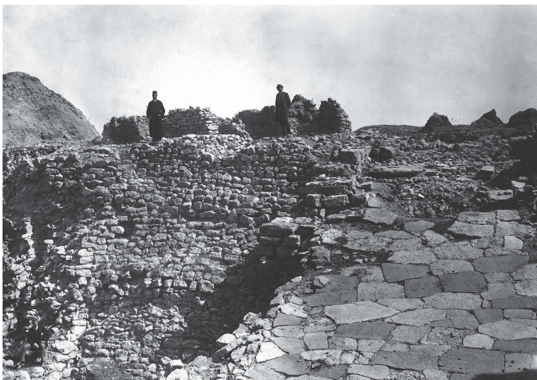
App. 7f Troy II fortification walls with ramp and gate FM (Dörpfeld photo 201).
